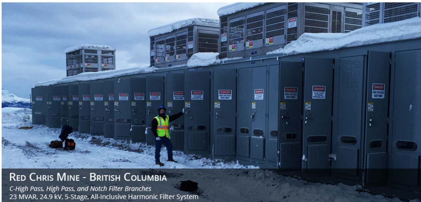
Figure 2 —Top, typical one-line diagram for a multi-tuned metal-enclosed harmonic filter system. All protection, disconnecting, switching and controls come preassembled, tested and ready for operation in a compact design from NEPSI. Picture is of harmonic filter system corresponding to one-line diagram.
