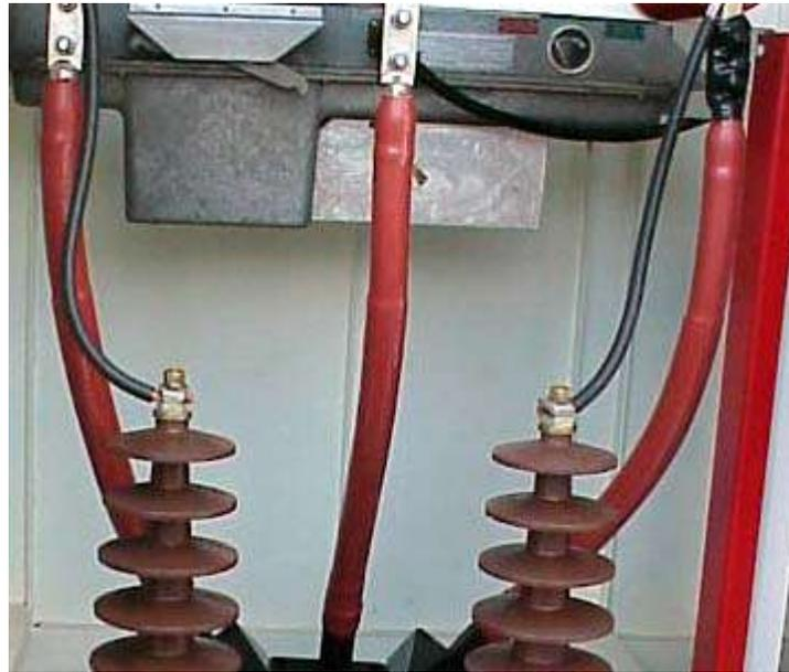
*Picture above shows a 34.5kV Raychem heat shrinkable termination installed in the incoming compartment of a 10 MVAR 34.5kV Harmonic Filter Bank.*
